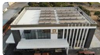
CHIA TAI Solar Rooftop 0.03 MW, 1 Sites 24 tCO 2 e
