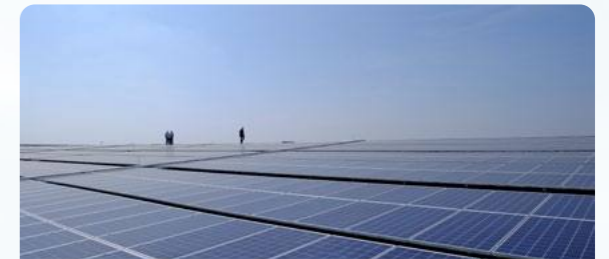
Total electrical power 197 MWP of sites with Solar PV installation
