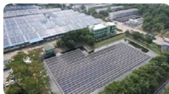
CPPC Solar Rooftop 4 MW, 1 Sites 3,256 tCO 2 e
