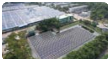
CPPC Solar Rooftop 4 MW, 1 Sites 3,256 tCO 2 e
